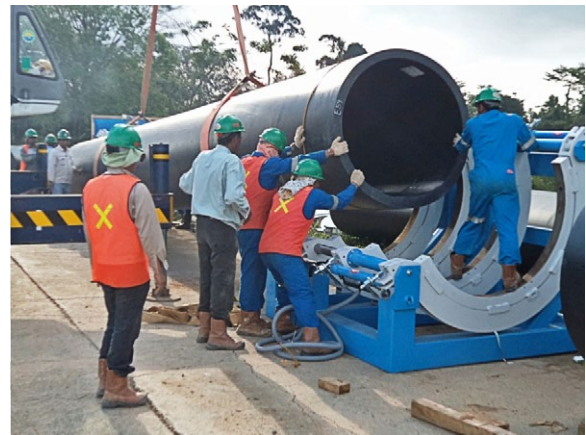
Figure 7: Welding on-site with a WIDOS 16000.
